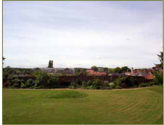
Figure 26 A vista of clay tiled roofs
