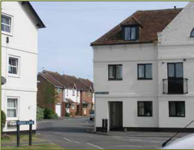
Figure 37 Modern windows in a historic building
