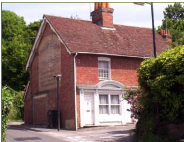
Figure 19 No 20/20A corner of Lode Hill and Slab Lane
