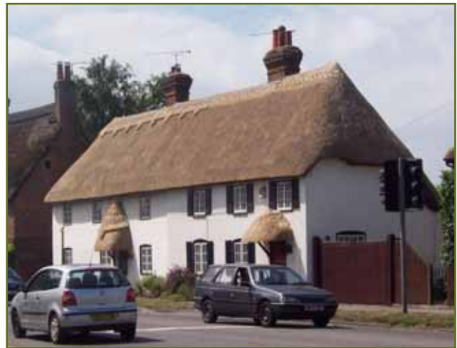
Figure 27 Simple traditional flush ridge on a thatched roof alongside block cut ridge
