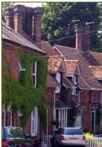
Figure 30 Chimneys at Waterside
