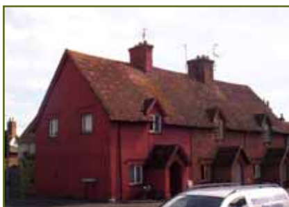
Figure 2 Distinctive porches (Nos 1-3 The Headlands)
