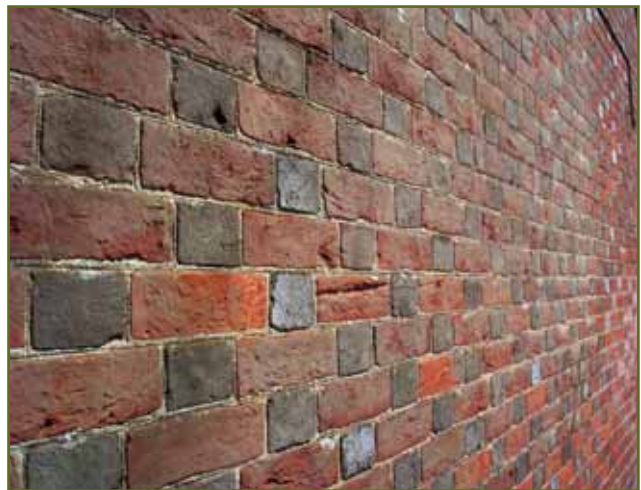
Figure 13 Flemish bond brickwork
