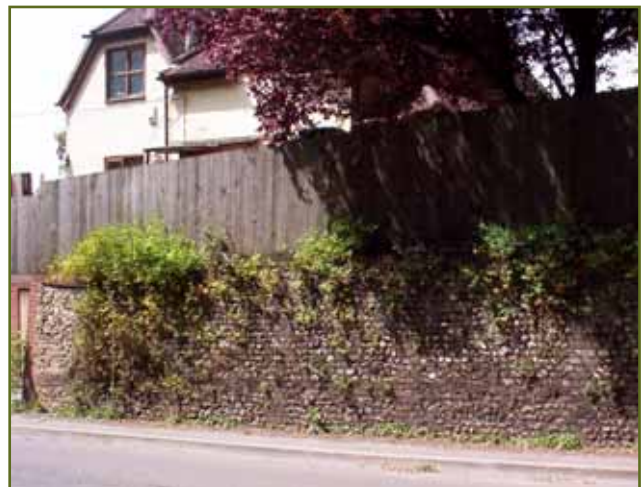
Figure 45 Flint wall Lode Hill
